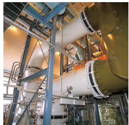
STENFLEX® type C-31 in a power plant
